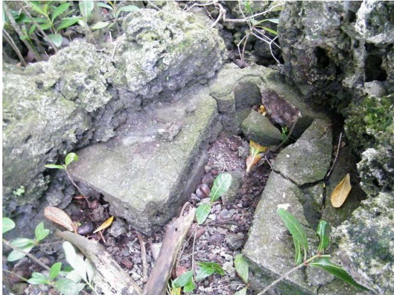
**Figure 4.17** AB176; a USMC concrete mount between coral rocks
