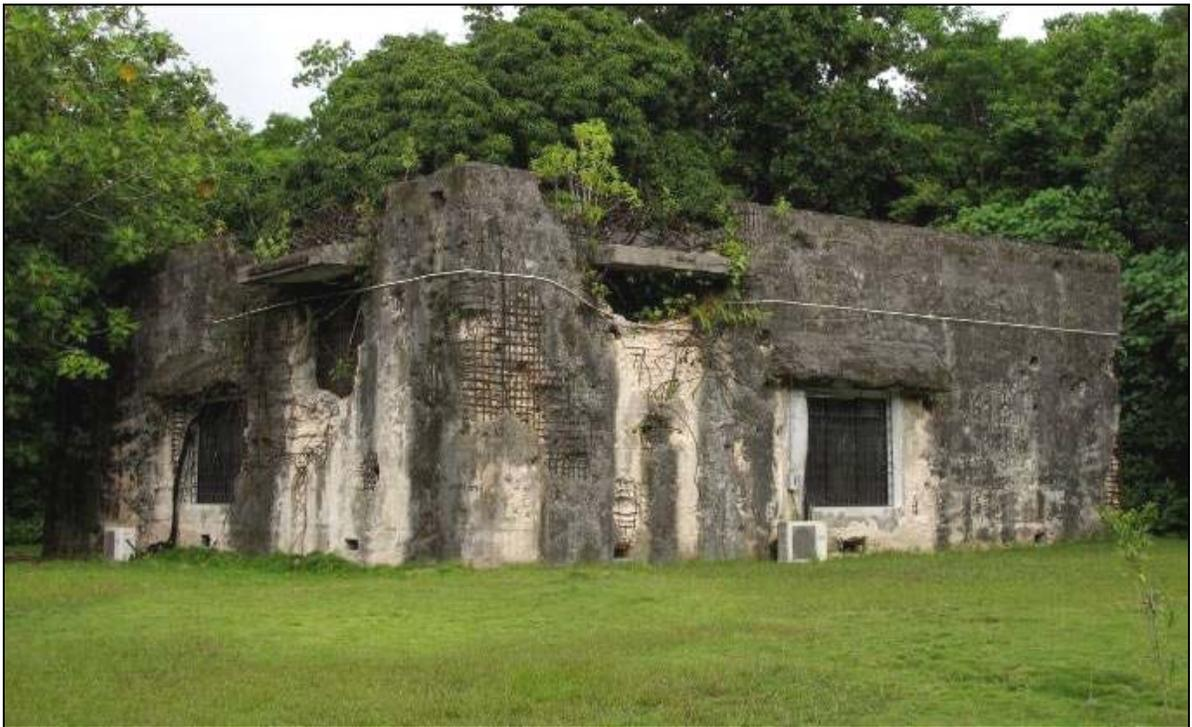
**Figure 3.26** AB168 in 2010, now a locally maintained WWII museum. The holes left by the 14 inch shells of American battleships have been covered and used as windows.
