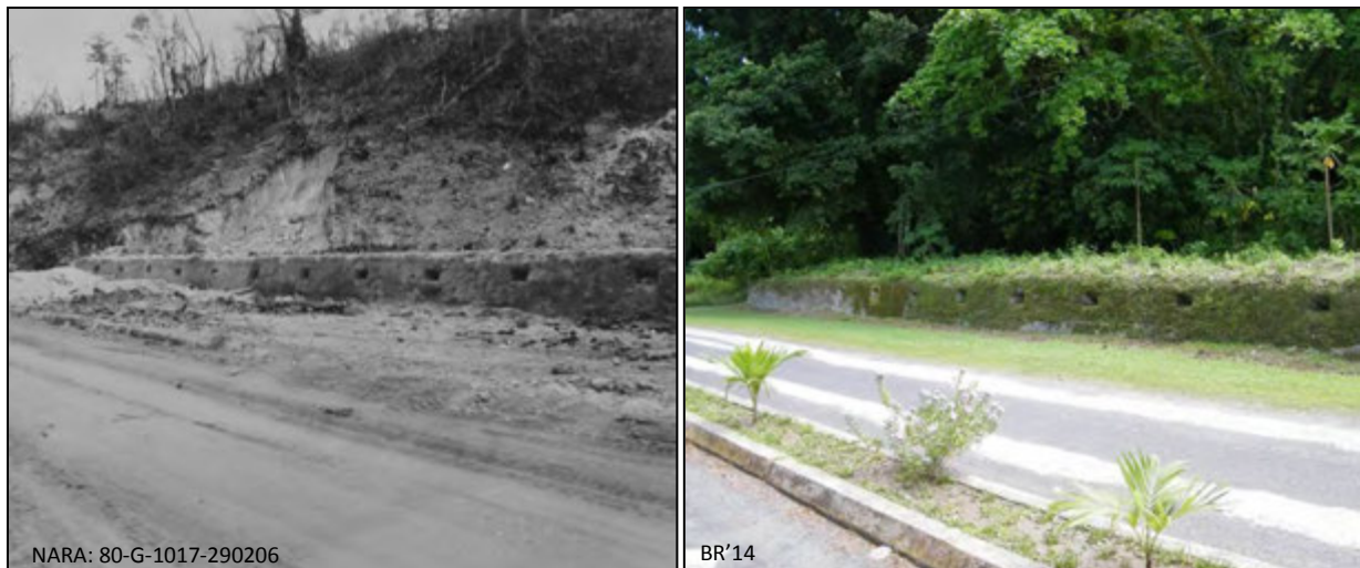
Figure 188 - AB155: converted Phosphate Drying Plant foundation slab; 18/12/1944 and 9/12/2014
