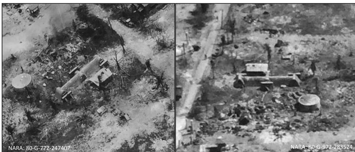
Figure 153 - AB14-107: north elevation 16/09/44 (left) and south elevation 26/10/44 (right)
