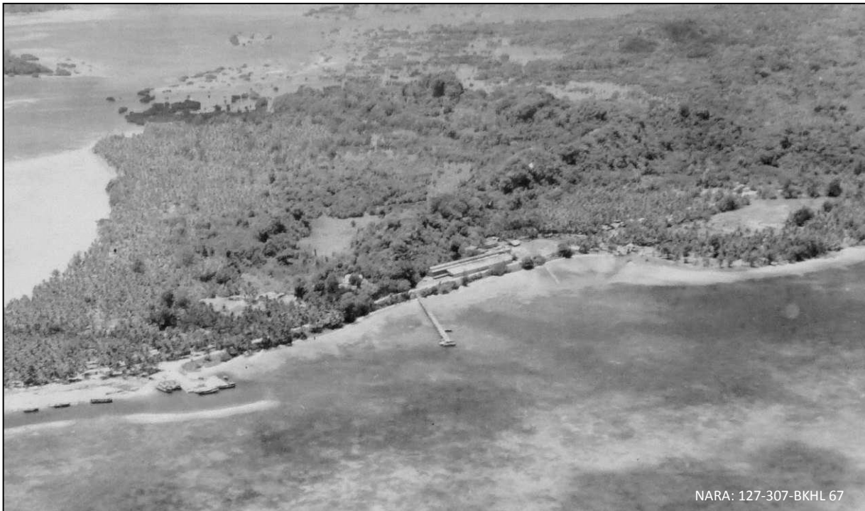
Figure 138 - Northern Peleliu on 31 st March 1944 showing the phosphate drying plant, loading pier and associated infrastructure
