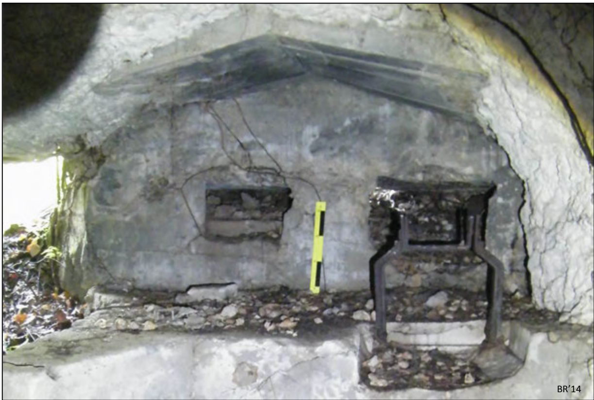
Figure 88 - AB14-109: interior view showing concrete and embrasures in south-east wall, October 1944 (above) and December 2014 (below)
