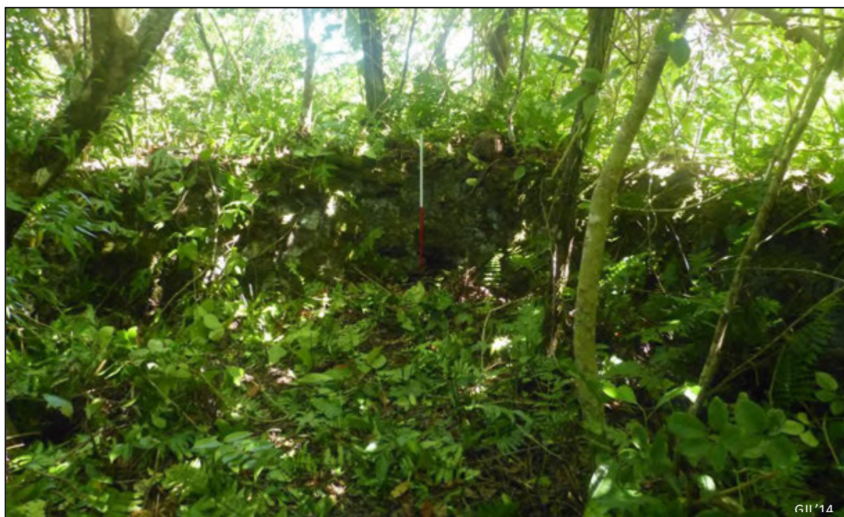
Figure 147 - AB14-070: interior view looking east showing rock cut parapet and flat base
