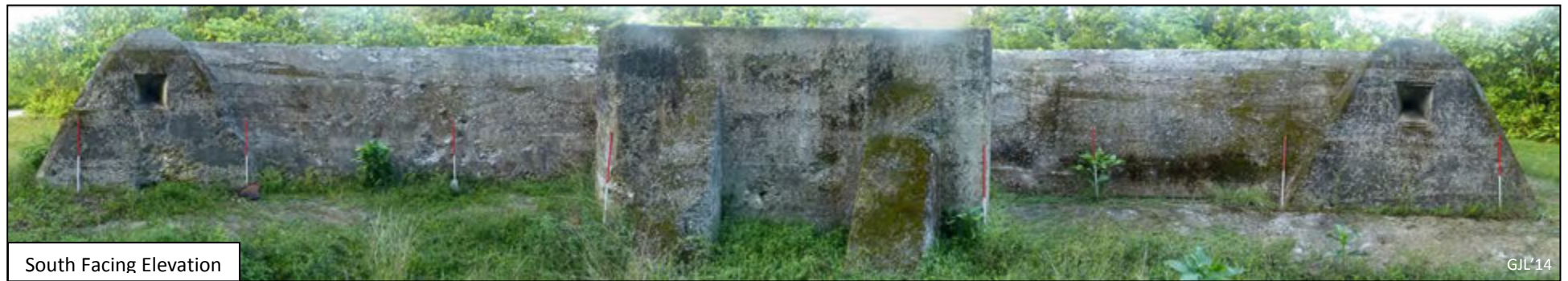
Figure 152 - AB14-107: photogrammetric survey of IJ air-raid shelter
