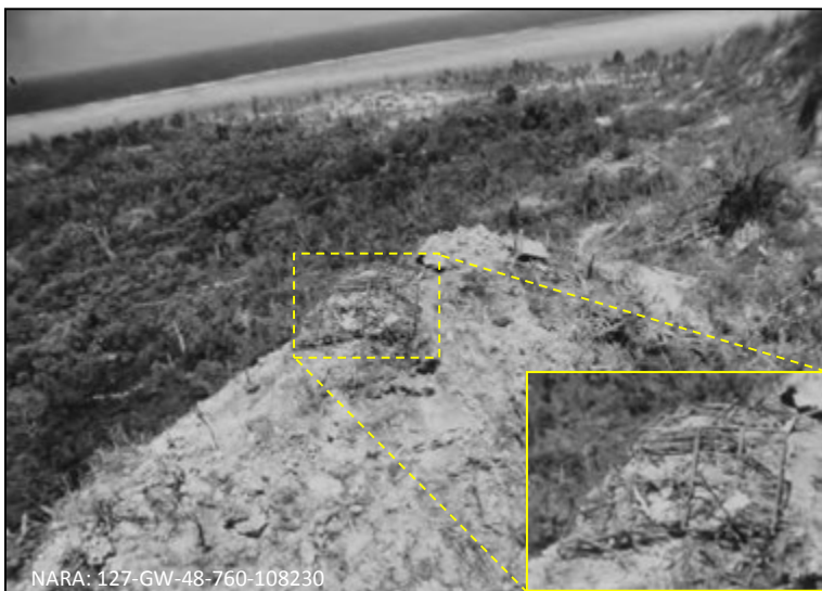
Figure 193 - Radar Hill with collapsed radar antenna
