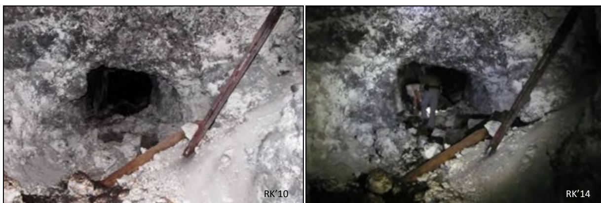
South passage at intersection looking north-west in 2010 (left) and 2014 (right)
