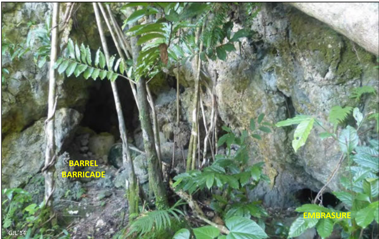
Figure 113 - AB14-054: entrance B showing concrete filled barrel barricade and rock cut embrasure
