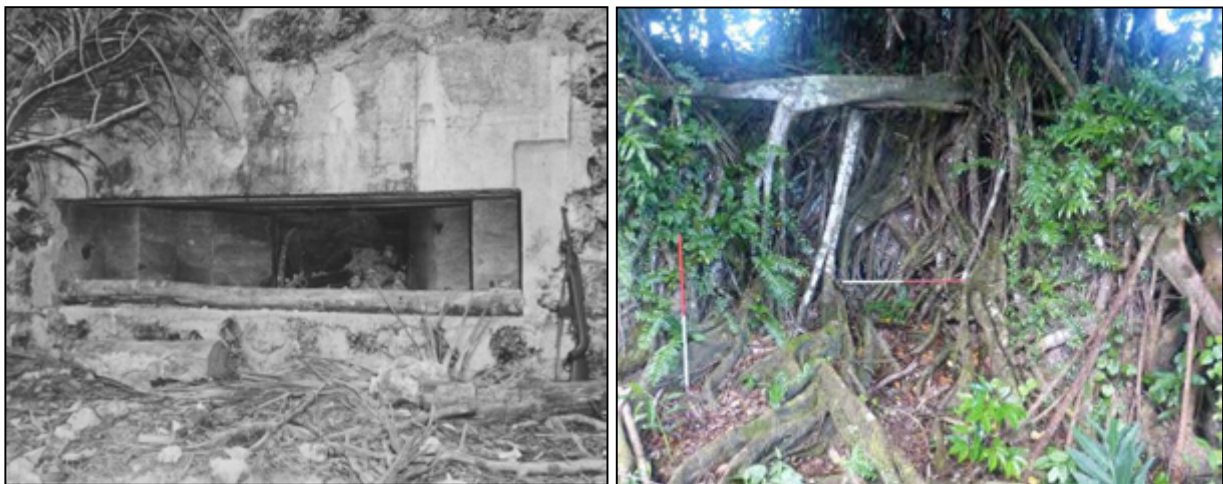
Figure 86 - AB14-106: west facing elevation showing main embrasure Oct.1944 (left), Dec.2014 (right)
