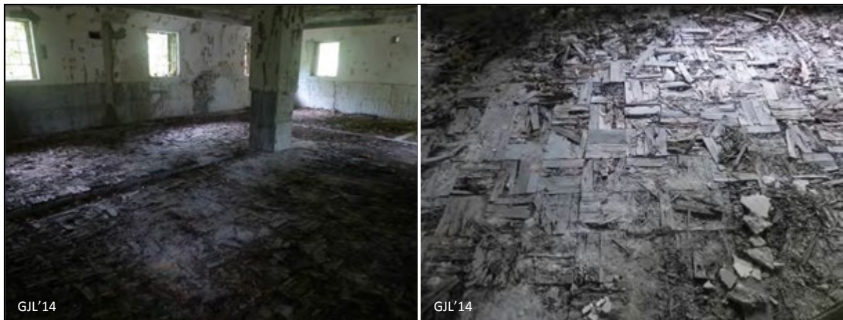
Figure 155 - AB38: second floor room showing detail of parquet flooring
