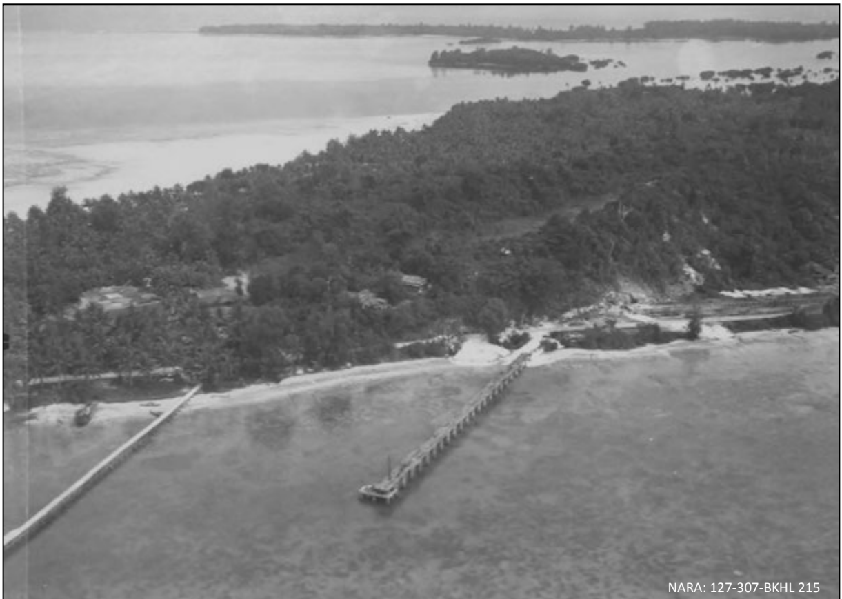
Figure 140 - Northern Peleliu on 25 th July 1944 showing demolished phosphate drying plant, loading pier and AB14-072 buildings on slope above
