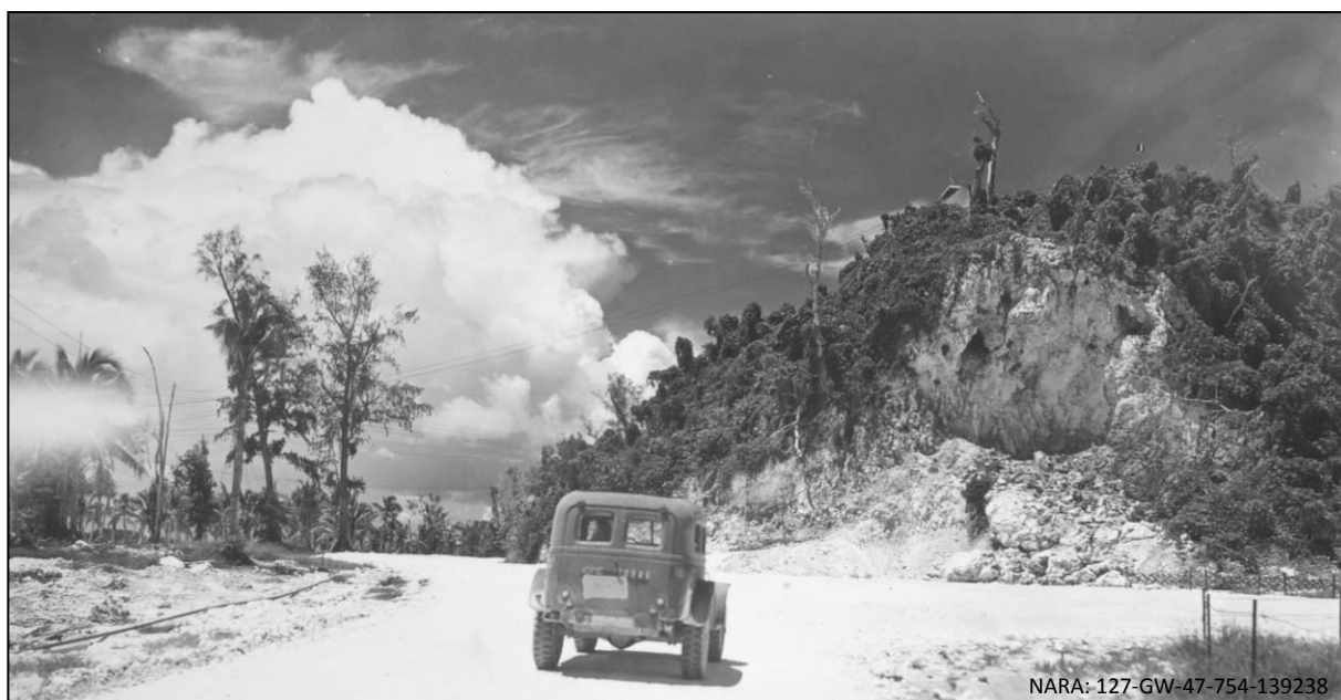
Figure 106 - The vertical face of Hill Row #1 showing evidence of the firepower used to reduce its concealed caves
