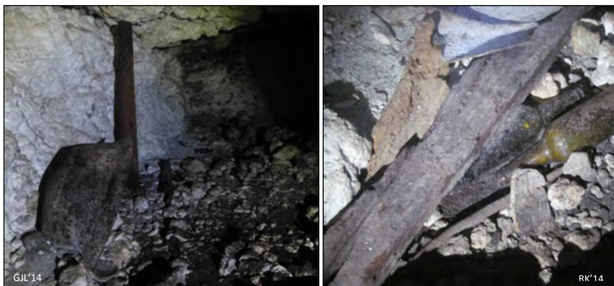
Figure 125 - AB14-063: main chamber showing in situ wall cladding timber and others collapsed across the floor
