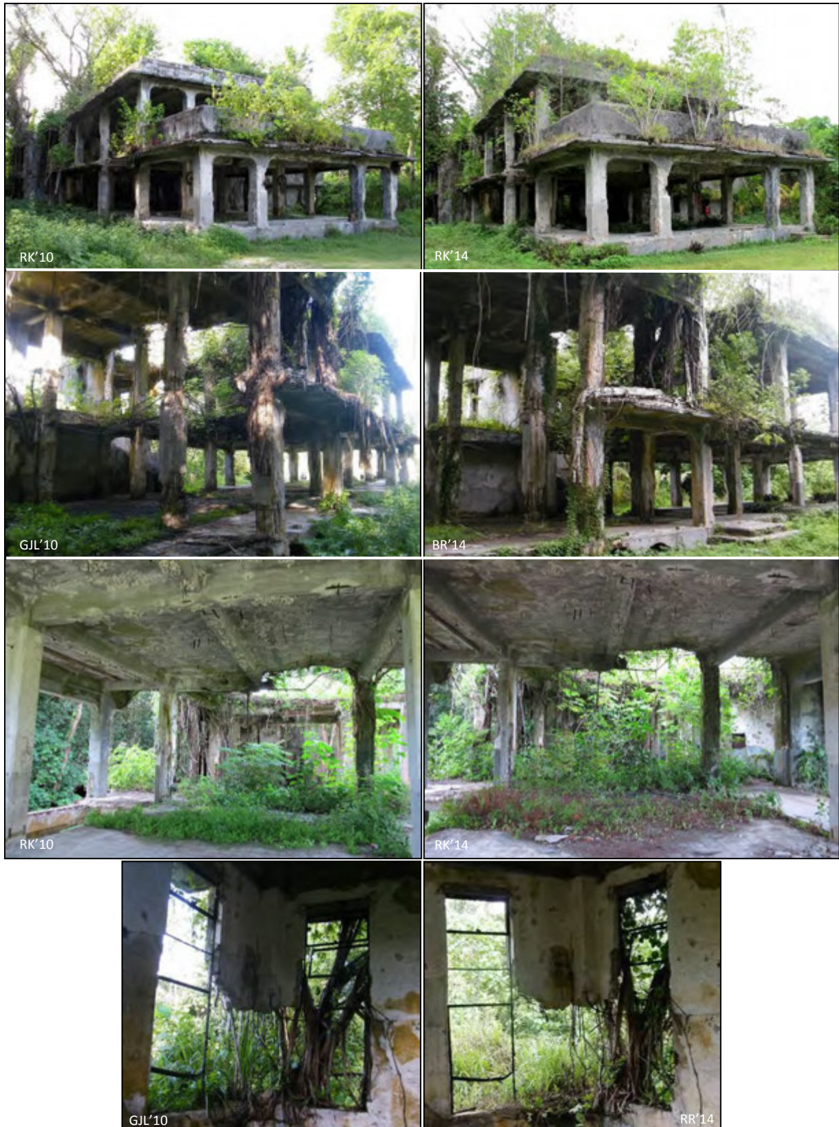
Figure 154 - AB38: Japanese Air Headquarters Building 2010 (left) and 2014 (right)
